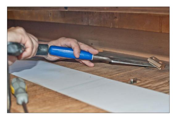
The old dag blocks held the old keyboard down against the keybed. Since you are replacing the keyboard, the old dag blocks serve no further purpose.
